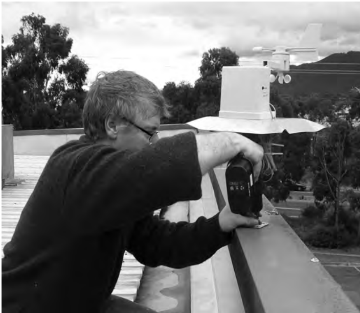
Figure 13-2. Weather station sensors and transmitter being installed
