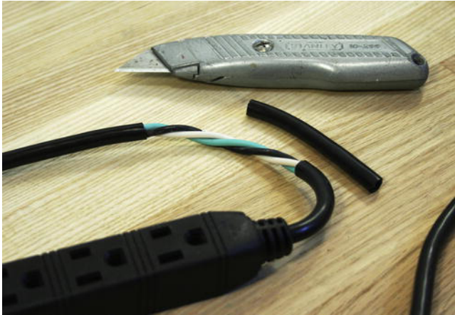
Figure 7-6. Outer insulation removed from power cable
