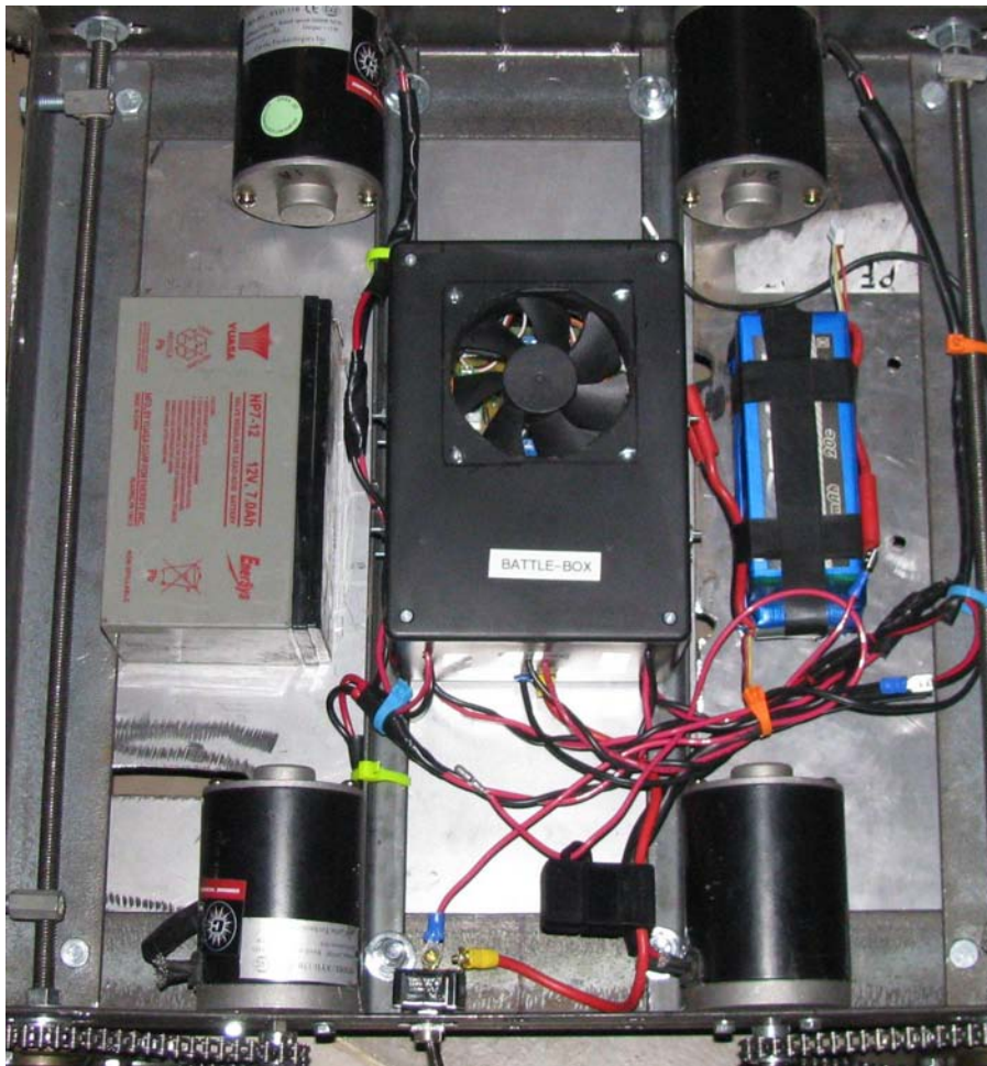
Figure 12-21. Either SLA (left) or LiPo (right) batteries fit in this frame.
