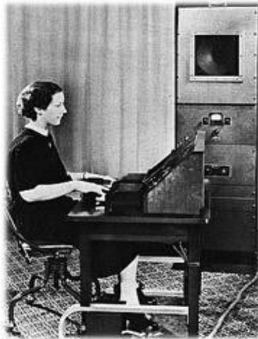
**Figure 16.20** The Voder developed by Homer Dudley of Bell Labs at the 1939 World's Fair in New York. The operator worked at a keyboard, with a wrist bar to control the voicing parameter and a pedal for pitch control.
