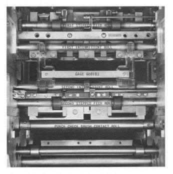
Figure 4-6. Gage Position in Punch Station
