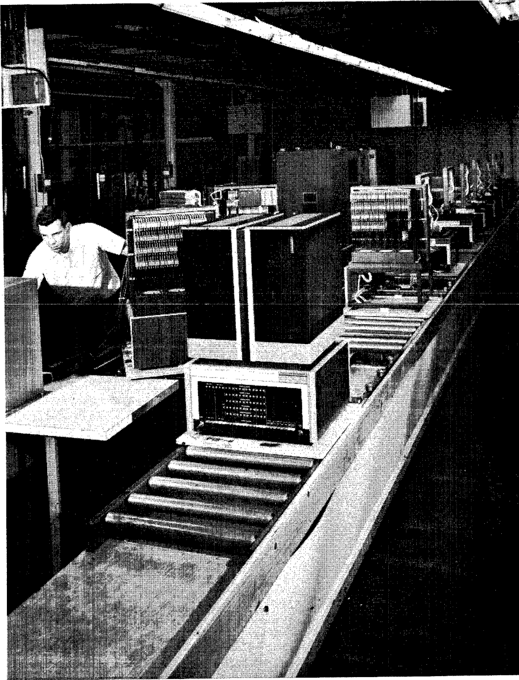
Digital's PDP-8 computer, shown here undergoing final production testing, is one of the most popular on-line computers for physics and biomedical analysis and process control.
