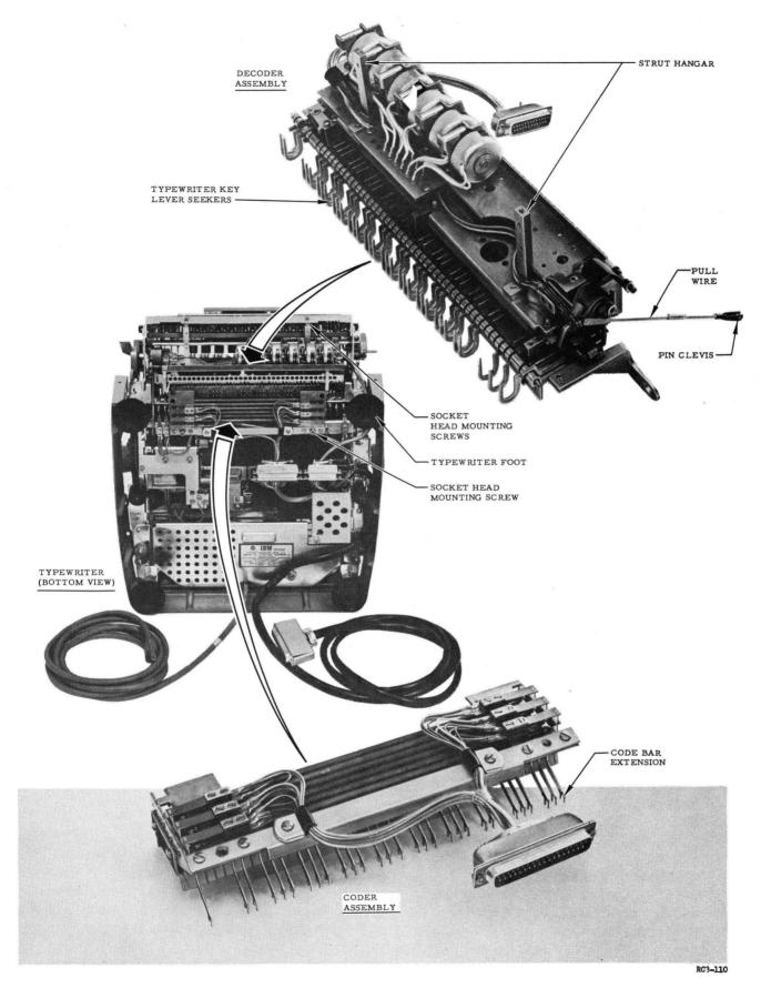
Figure 31. Coder and Decoder Assembly and Removal
