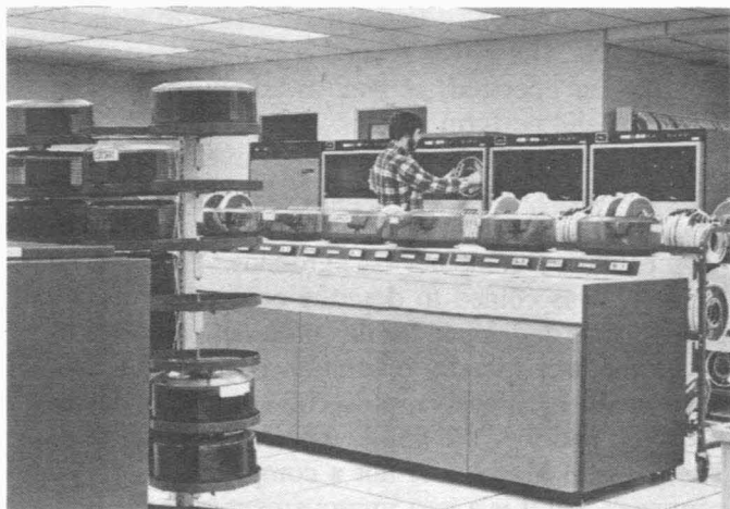
Fig 1.1 A modern mainframe computer center
