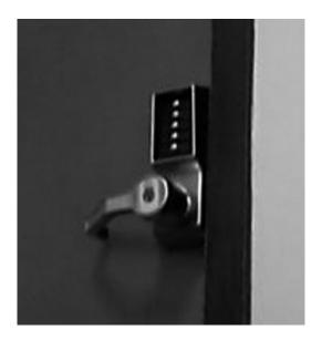
Noted security researcher Michal Zalewski goes high-tech against locks like this and his results are nothing short of spectacular. In his paper "Cracking Safes With Thermal Imaging" (http://lcamtuf.coredump.cx/tsafe), Michal shows that heat left behind from a user's fingerprints can be detected with a thermal imaging device up to several minutes later, as shown below.
