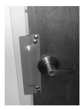
OK, so that's more of a door *chasm*, and it wouldn't take much to get a finger in there, if it weren't for that clever security device (the steel plate) covering it. The plate does solve the credit card problem, but as you can see from the next photo (shot looking down inside the door gap at the latch mechanism) the gap is so ginormous that another type of tool could be used to bypass the door.
